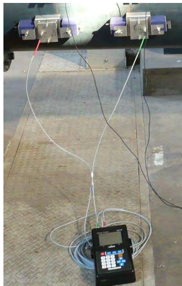
Fig. 1.2.9-56 Setup is completed
