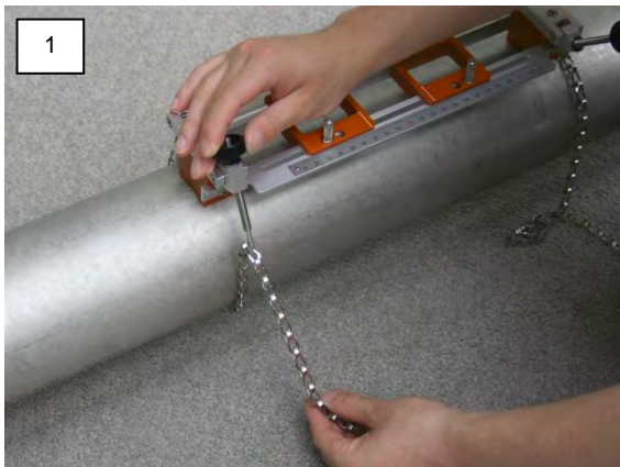
1. Roll chain around the pipe.
